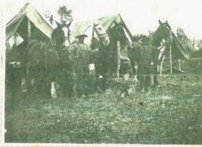
CONSTRUCTION CREW WORKING ON THE OSTERUND ROAD 1918
